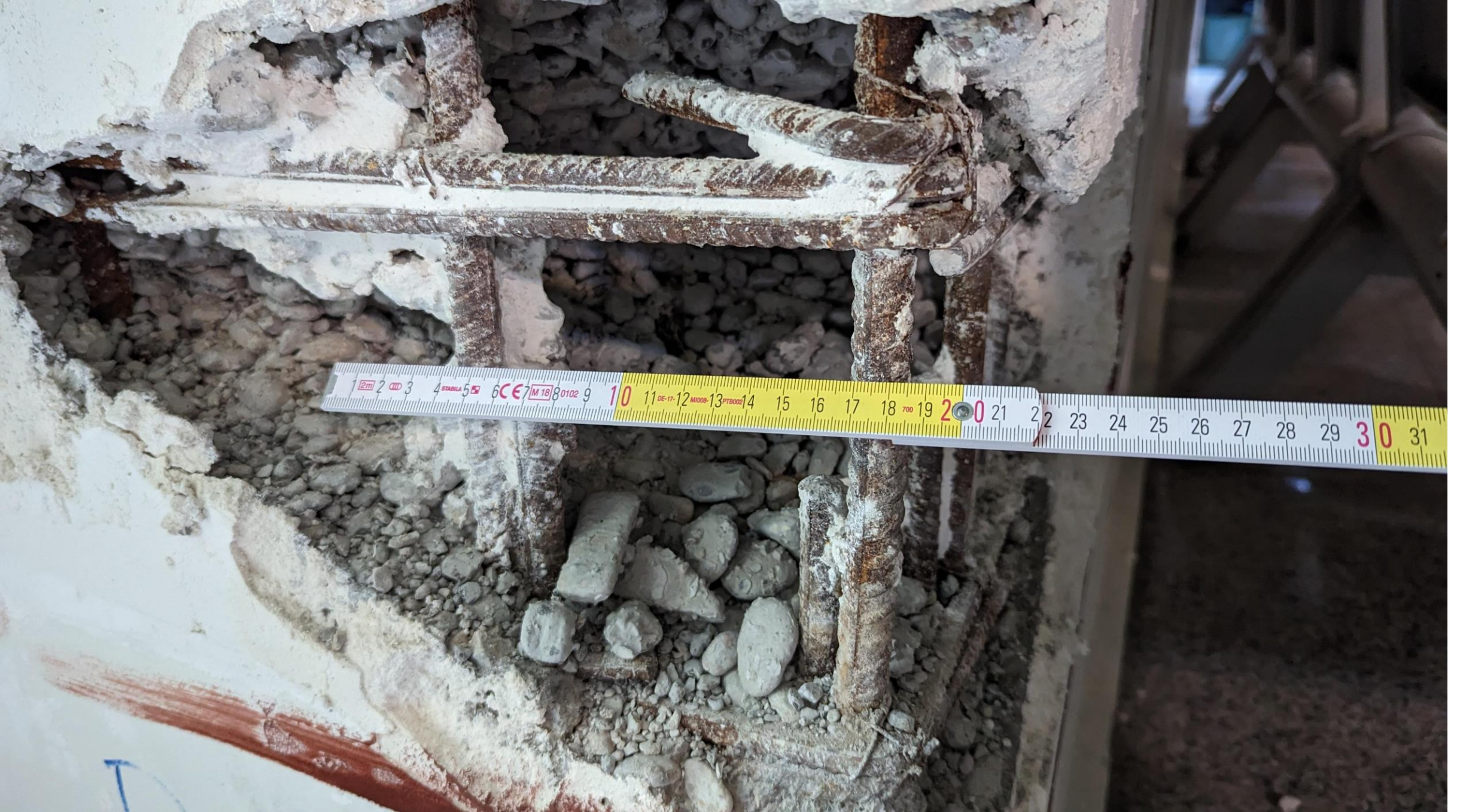
2023-04-24 Necip Fazıl City Hospital 市立醫院
